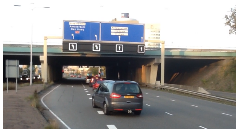
Figure 2-2: Dynamic message signs indicate the lane use at the intersection A12–Europalaan in Utrecht
