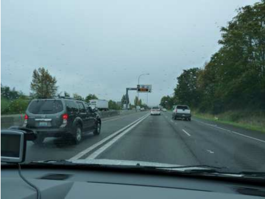
Figure 18: HOT Lane in Seattle
